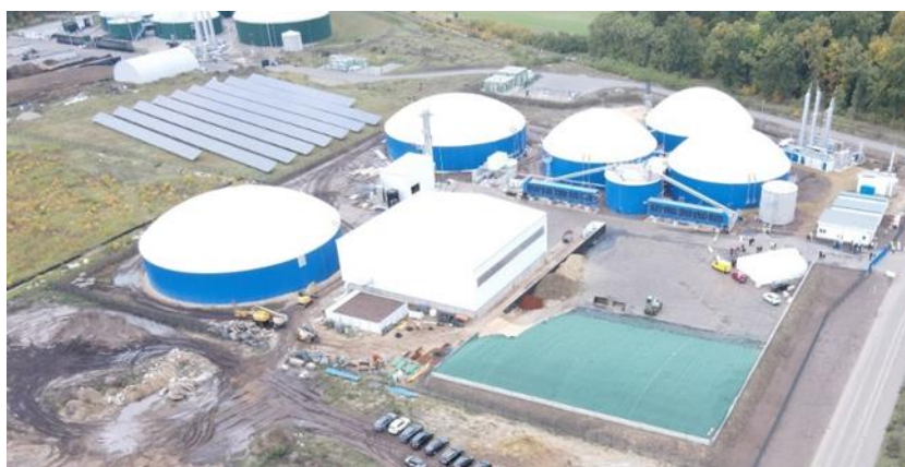
Figure 7-12 Biogas plants built in different parts
